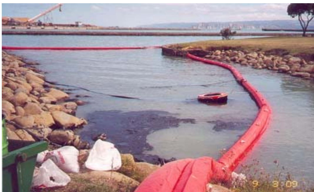
Figure II. Booms for containing an oil spill
