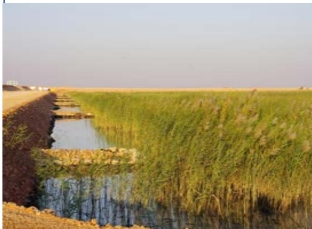
Fig. 9. Reed beds for produced water purification in Oman 50
