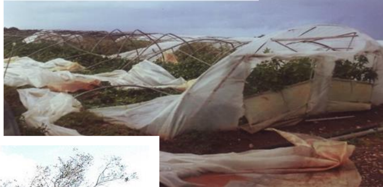
Storm effects on Greenhouses, 19/1/2018
